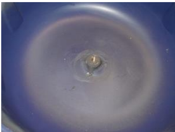
J B Weld filled cracks
